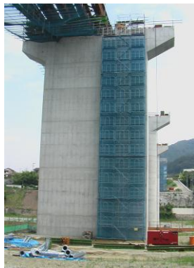
Figure 2. Modern scaffolds used in construction sites.
