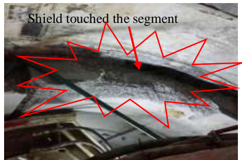
Figure 4. Crack at front part of the segment due to lack of clearance.
