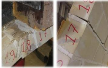
Figure 1. Cracks on the masonry vaults *ante operam*.
