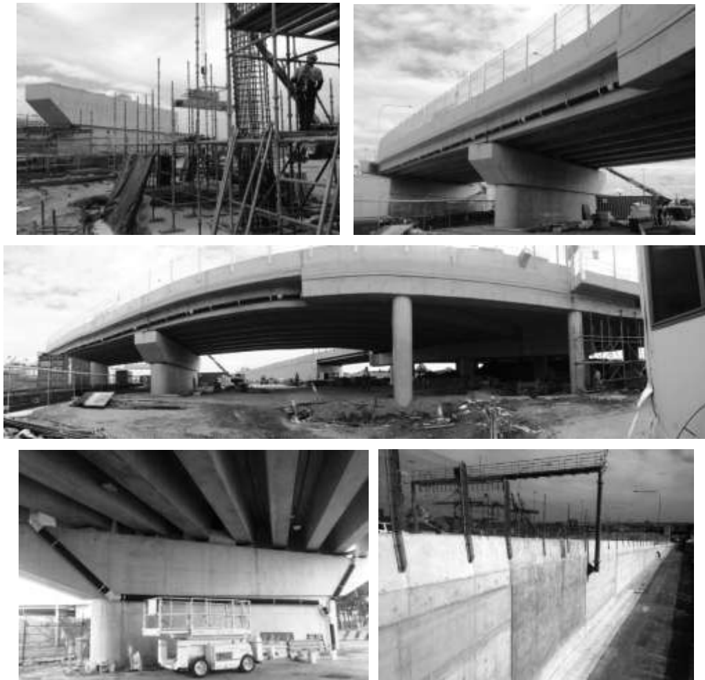
Figure 1. Ramp D Construction Photos (photos by author).
