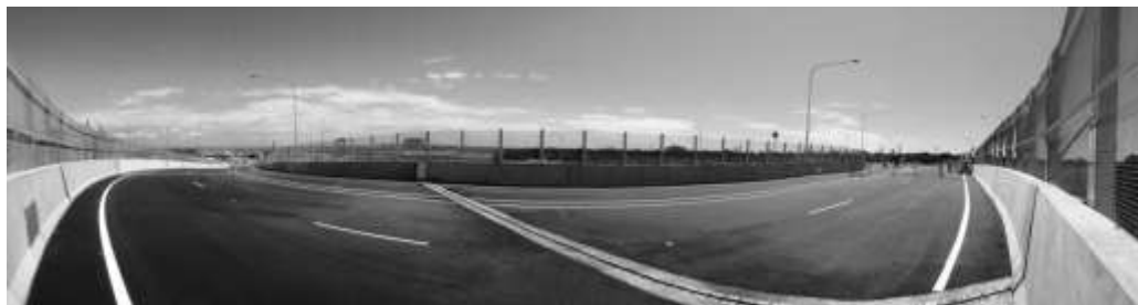
Figure 2. The Completed Ramp D (photo by author).
