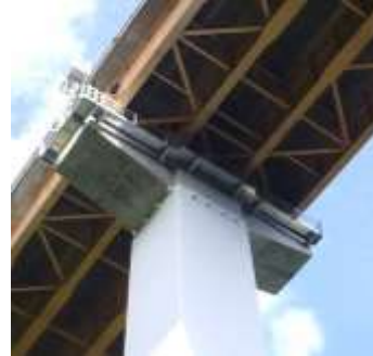
Figure 4. Strengthening of column by steel plate jacketing.
