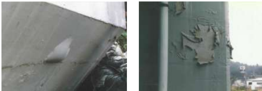
Figure 2. Breaking of the epoxy coating due to trapped residual water.
