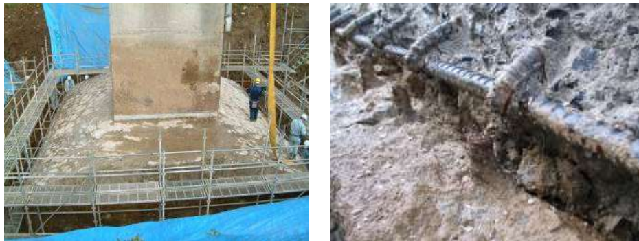
Figure 1. Fracture of rebars and surface cracking on the footing of a bridge.
