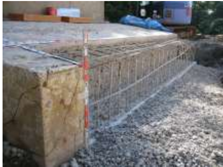
Figure 3. Partial reconstruction of bridge footing with fracture of rebars.
