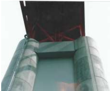
Figure 5. Strengthening of column by immersed PC confined method.
