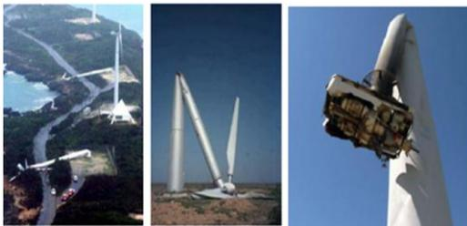
Figure 1. Buckling failure of steel tower.
