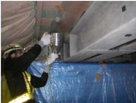
Figure 3. The spraying operation.
