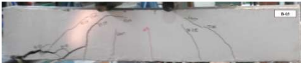
Figure 7. Failure mode of beam with vertical strengthening.
