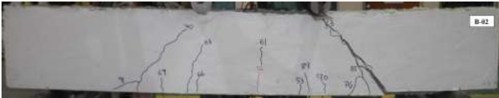
Figure 6. Failure mode of beam with horizontal strengthening.
