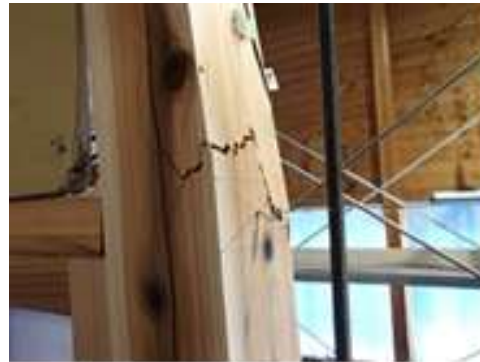
Figure 10. Column damage on the plus side in specimen 4.
