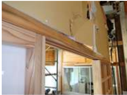
Figure 11. Deformation of plaster board in the out-of-plane direction in specimen 4.
