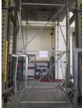
Figure 8. Failure of Spec. 2L-D48A-2.
