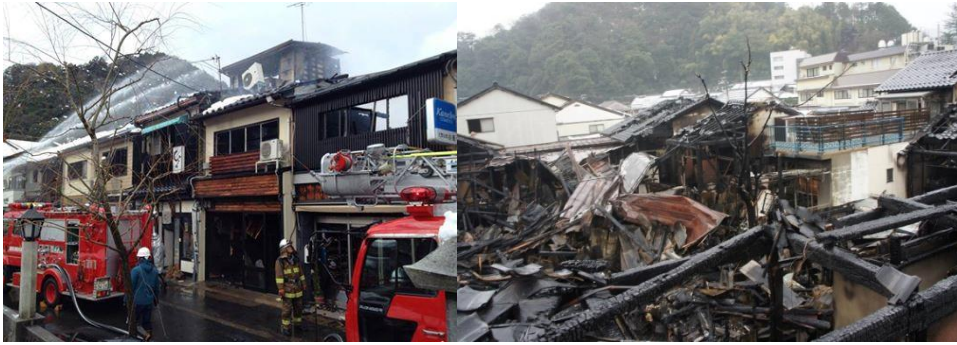
Figure 1. Fire spreading site at Kinosaki Spa resort area (Kobe Newspaper 2015).
