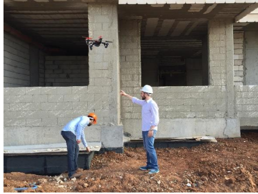
Figure 4. Drone capturing videos on construction site.
