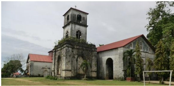
(a) Southeastern part of church before Bohol earthquake
