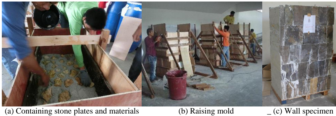
Figure 4. Construction of wall specimens.
