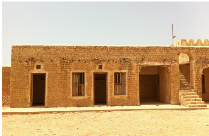
Figure 3. Al Thagab Fort, the external walls are constructed with layers of alternated coral rock and limestone blocks having a regular shape (Source: Author).
