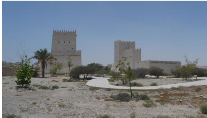
Figure 2. The Barzan Towers in Doha. The restoration works recently completed (Source: Author).
