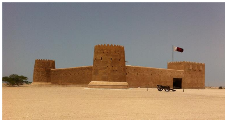
Figure 1. Al Zubarah Fort, the restoration works recently completed (Source: Author).
