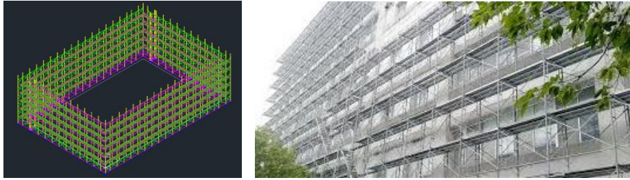
Figure 6. Scaffold for the building.
