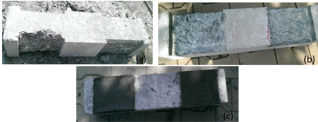
Figure 1. a) Side face chipped off beam (Stage 1); b) Epoxy layer applied after chipping off (Stage 2); c) Beam retrofitted with UHP-FRC (Stage 3).
