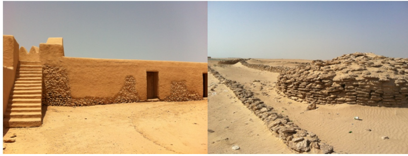
Figure 1. Left: Al Rekayat Fort, the circular tower on the corner. Right: Bir Zikrit Fortress and the current state of conservation of the defensive wall's ruins.
