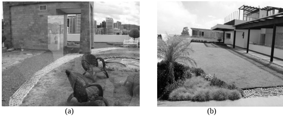
Figure 1. a) Green roof at the Ministry of the Environment building in Quito; b) one of the green roofs at the vivAlto building.
