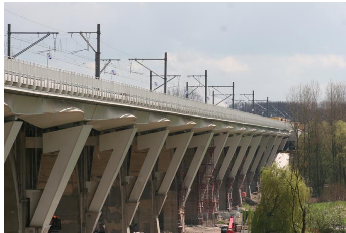
Figure 4. Earlier expansion works on the Pede viaduct.
