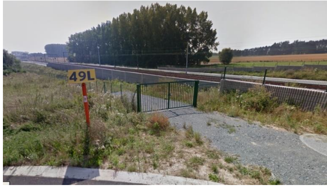
Figure 2. Ballast walls for the Borrestraat bridge.
