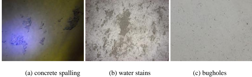
Figure 1. Typical degradations in tunnel lining concrete.
