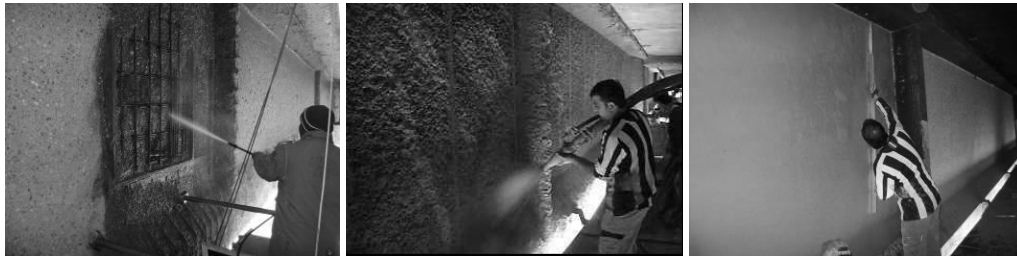
Figures 3, 4, & 5. Different stages of repair work.
