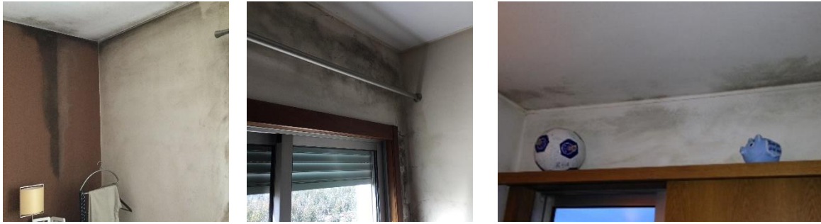
Figure 2. Examples of observed anomalies (condensation, humidity).
