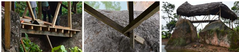
Figure 7. Foundation of the bridge, roof structure of Bolivar's Lookout.
