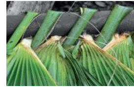
Figure 6. Toquilla straw roofing.
