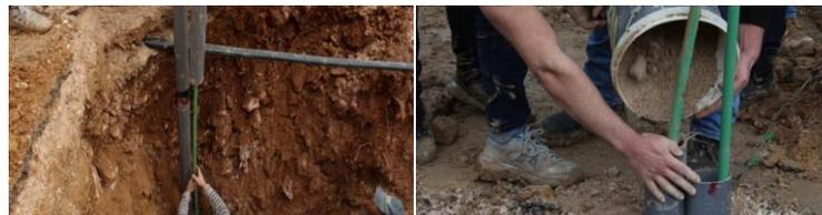
Figure 4. Connecting the pipe network in the asphalt layer with that in the soil.
