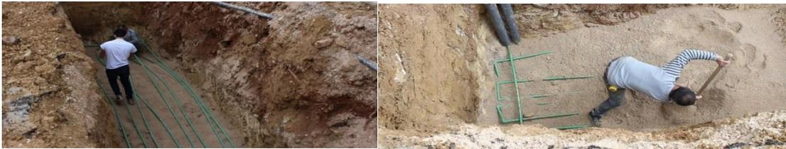
Figure 3. Placing fine material below and above the pipes.
