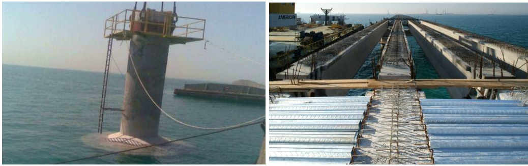
(a) Precast pier columns.
