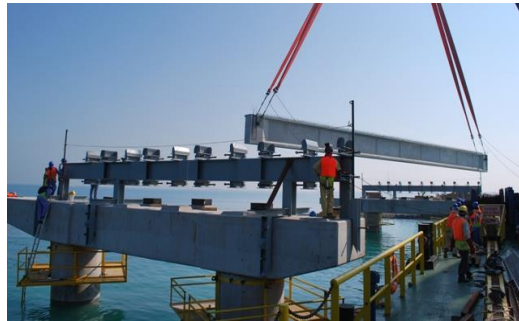
Figure 3. 2.2 m deep, 39.6 m long AASHTO girder.
