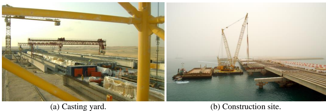
Figure 4. Fabrication and erection of precast girders.
