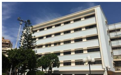
Figure 1. Beirut Arab University Block C eastern facade.
