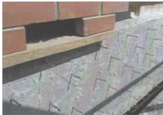
Figure 6. Mesh of mechanical pinning and remedial tying system “DryFix”.
