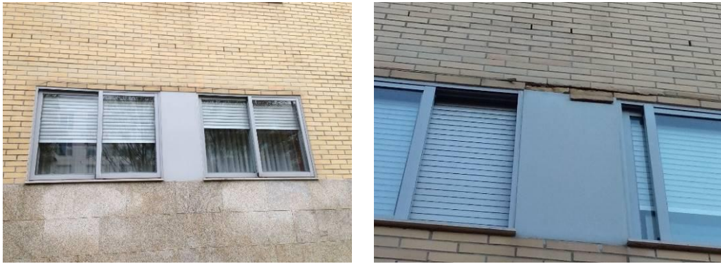
Figure 3. Horizontal cracks of the lintels.
