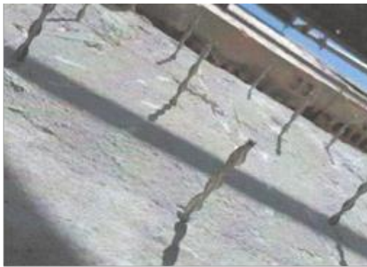
Figure 5. Bottom view of the support of the exterior coating of the masonry double wall.
