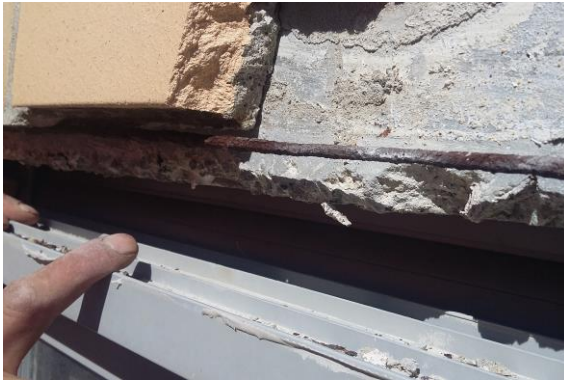
Figure 8. Existent iron rod in cracked lintels.
