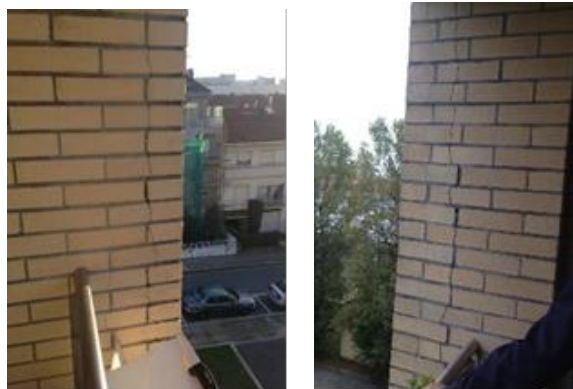
Figure 4. Vertical cracks of the brick wall-corners balconies.
