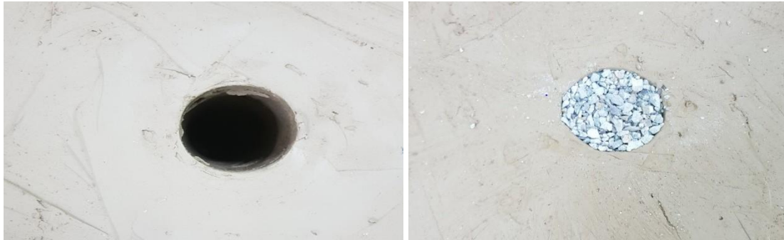
Figure 4. Stone column installation.
