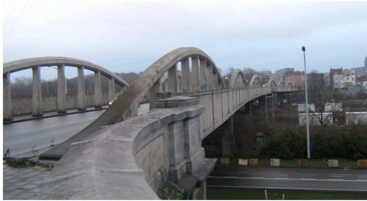
Figure 1. Six span concrete arch bridge Rampe du Lion.
