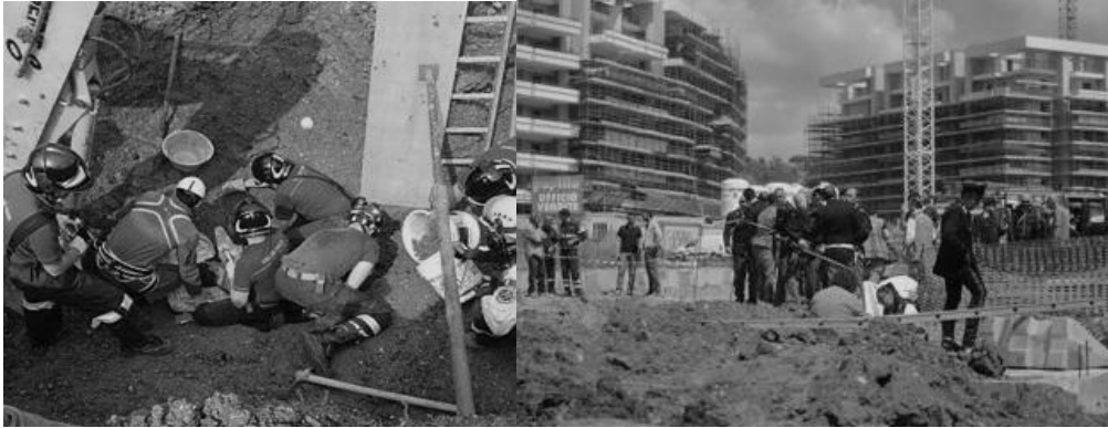
Figure 1. Excavations in the trenches. Incidents in the year 2014 on construction sites in Turin and Rome.
