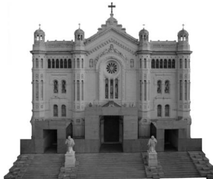
Figure 4. The provisional structure built to protect the entrances.
