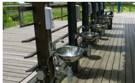
Figure 4. Hydro-powered Sensor Water Taps.
