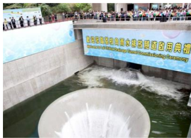
Figure 3. Novel drainage tunnel to mitigate effect of flooding due to extraordinary rainfall.
