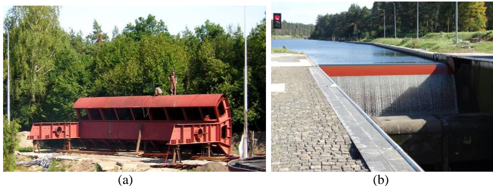
Figure 2. A view of the sluice flap: a) before mounting, b) after mounting.
