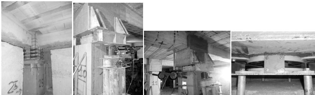
Figure 7. Images of the works performed for the base-isolation of the building.
