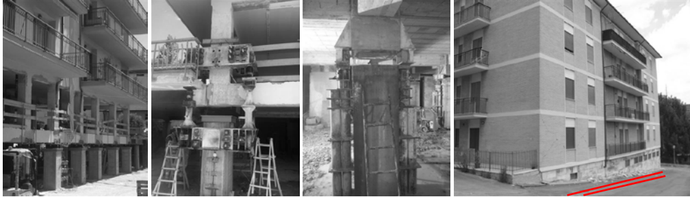
Figure 1. Buildings retrofitted through base isolation.
