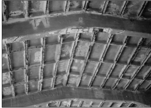
Figure 1. Reinforced concrete roof elements: cracking and spalling of concrete cover; uncovering of the steel reinforcements.
