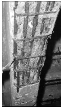
Figure 2. Reinforced concrete beam: advanced corrosion of the steel reinforcements, reduction of the diameter and fracture of the stirrups, in some areas, due to the corrosion by chloride ions.
