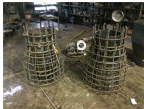
Rebar and inner tube
