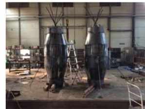
Fabrication of segment
