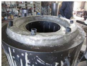
Shear key and sheath tube
