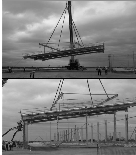
Figure 5. Lifting and fixing of the pre-assembled roof panels.
