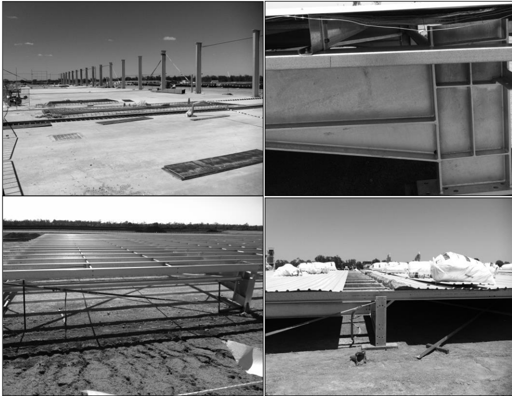
Figure 4. Roof panels assembled on the ground.
