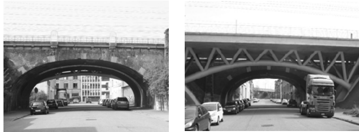
Figure 1. The existing MSB before refurbishment ( right ); the new MSB for the high-speed railway line ( left ).
