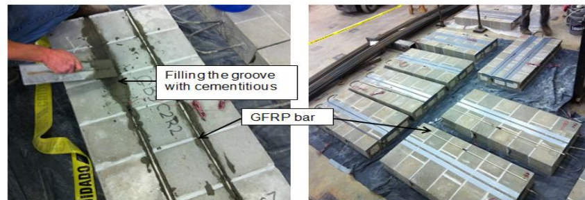
Figure 1. Installation of FRP bars in grooves.
