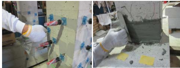
(a) Rebuilding of damage cross section with PCM (b) Injection of epoxy resin
