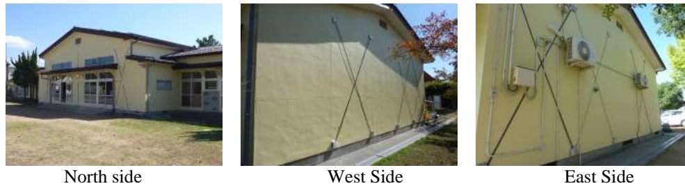
Photo 1. View of one-story kindergarten wooden structure retrofitted with “BRACE-X”.
