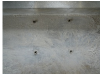
(b) Installation of mechanical.
