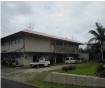
Picture 1. Appearance of the building.
