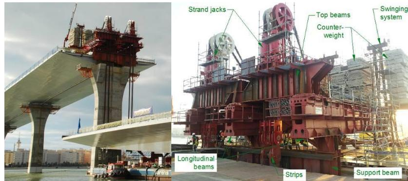
Figure 5. Lifting frame installed in pier P9. The picture at the left shows the deck already installed.
