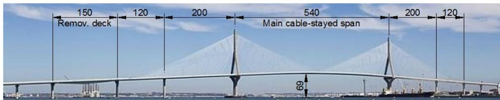
Figure 1. General elevation of the viaduct over the Cadiz Bay.
