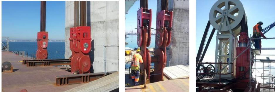
Figure 4. Strips connected to the deck (left) and strand jacks of a lifting point (right).
