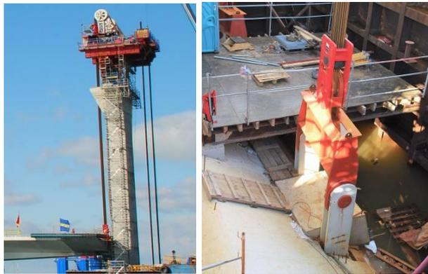
Figure 6. Lifting frame installed in pier P10 (left) and anchorage to the pier cap (right).
