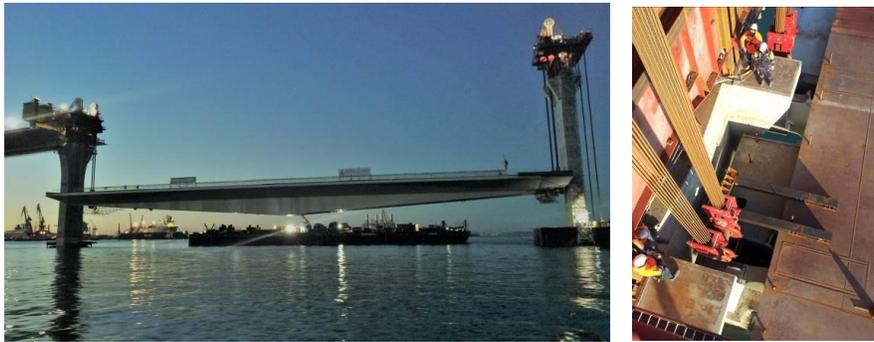
Figure 7. Starting of the lifting (left) and the deck passing through the corbels (right).
