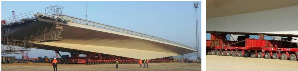
Figure 2. General view of the land transportation with SPMTs (left) and the transporter beams (right).
