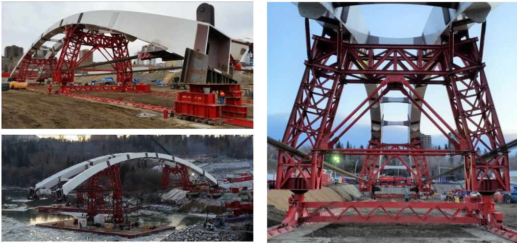
Figure 2. Skidding and load-out of the 1,000 T arch.
