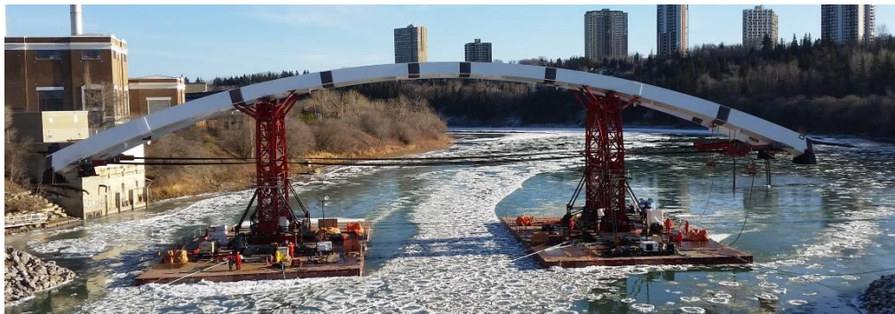
Figure 3. Navigation of the 1,000 T arch with two modular barges and eight winches.
