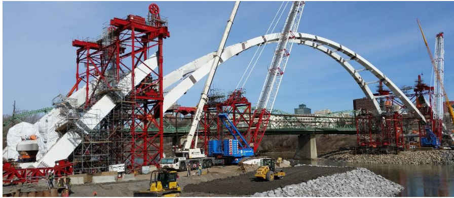
Figure 5. Lifting 20.5 m of the 1,800 T arch by means of four strand jacks.
