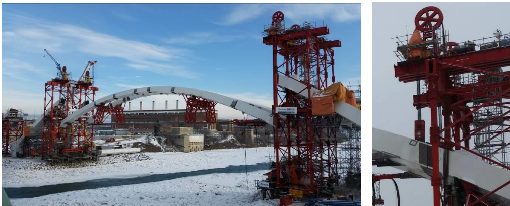
Figure 4. Lifting 15.5 m of the 1,000 T arch by means of four strand jacks.
