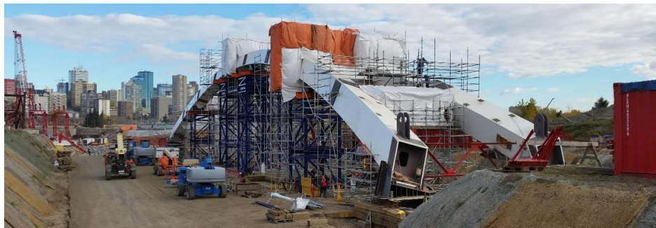
Figure 2. Central arch (1,000 T) being manufactured on temporary supports.
