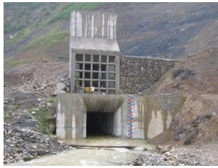
Figure 5. The diversion tunnel.
