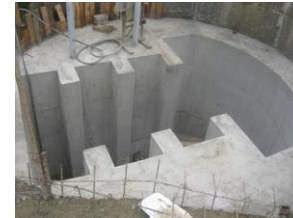
Figure 10. Vertical shaft of intake structures.
