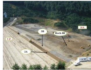
Figure 6. The dam body cross-section.
