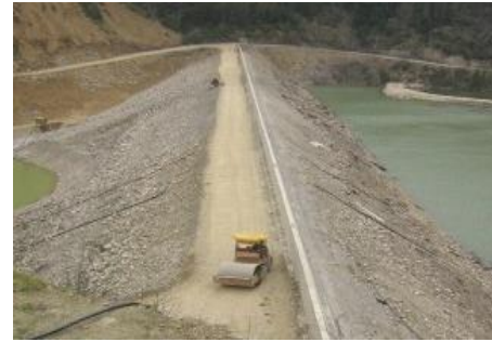
Figure 4. Upstream Cofferdam.
