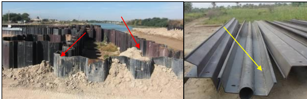
Figure 2. PPM and Installation of sheet piles walls near the cell dam workshop (Turk 2004).
