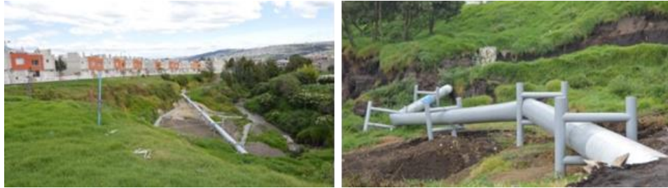
Figure 6. Project site (Sanshayaku Gully), before and after.
