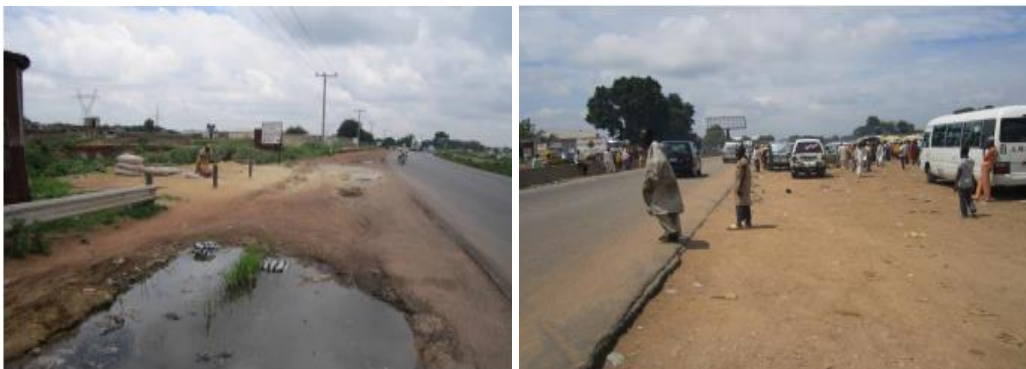
Figure 1. Some samples from observed hazardous features along the studied road sections.
