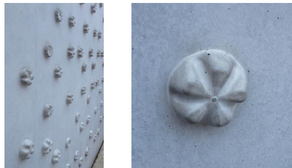
Figure 1. SCC-wall of the Vorarlberg Museum in Bregenz, Austria.
